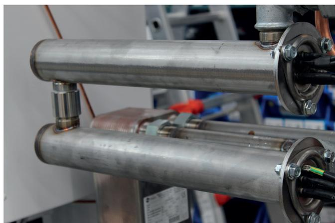
The function AES for the units HC allows the recovery of the fluid from the utility and shall be combined with the installation of an expansion tank on the centralized water line.
